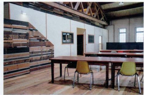
The interior of the Green Garage illustrates some of the make-do design approach so prevalent in the D. The space incorporates reclaimed and recycled pipes, wood and bricks from its previous incarnation as well as material salvaged from a nearby defunct Cadillac dealership and Detroit brick manufacturer. Photo: Michelle and Chris Gerard.
